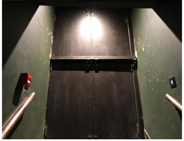
Photo taken @ 01:50hrs – 2<sup>nd</sup> August 2020. Side fire exit from basement floor of Mahiki to Southmill Street. Locked, bolted top and bottom and secured with a steel bar.
